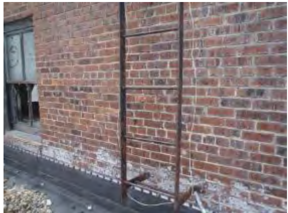
Ladder on Roof
