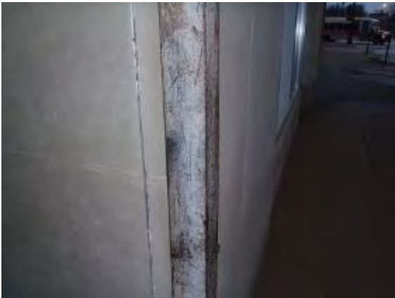
Corner Guard NW Corner
