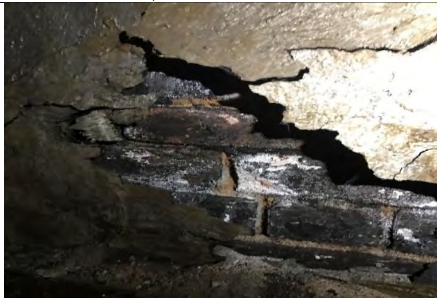
Samples 139-141 – Boiler Wrap – Tar
