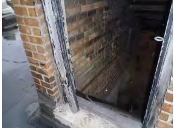
Door Components on Roof
