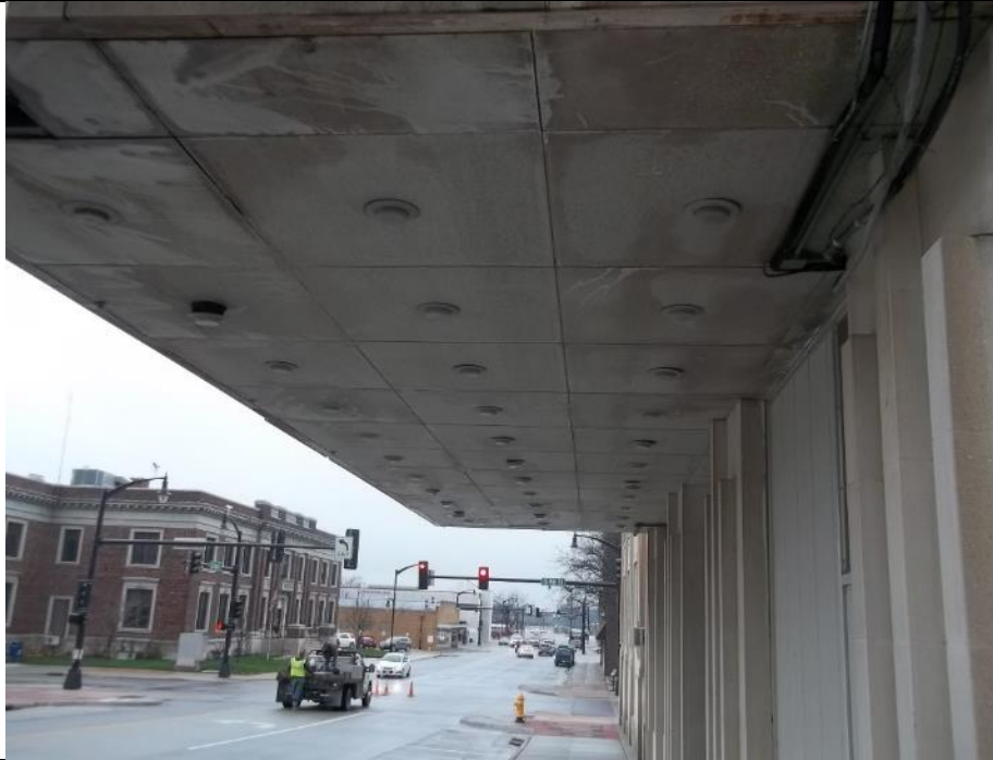
Sample 90 - Transite Soffit over entrance on 1 st Ave S.
