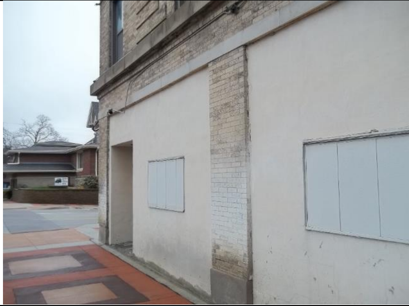
Samples 204 – Caulking around smooth stucco siding
