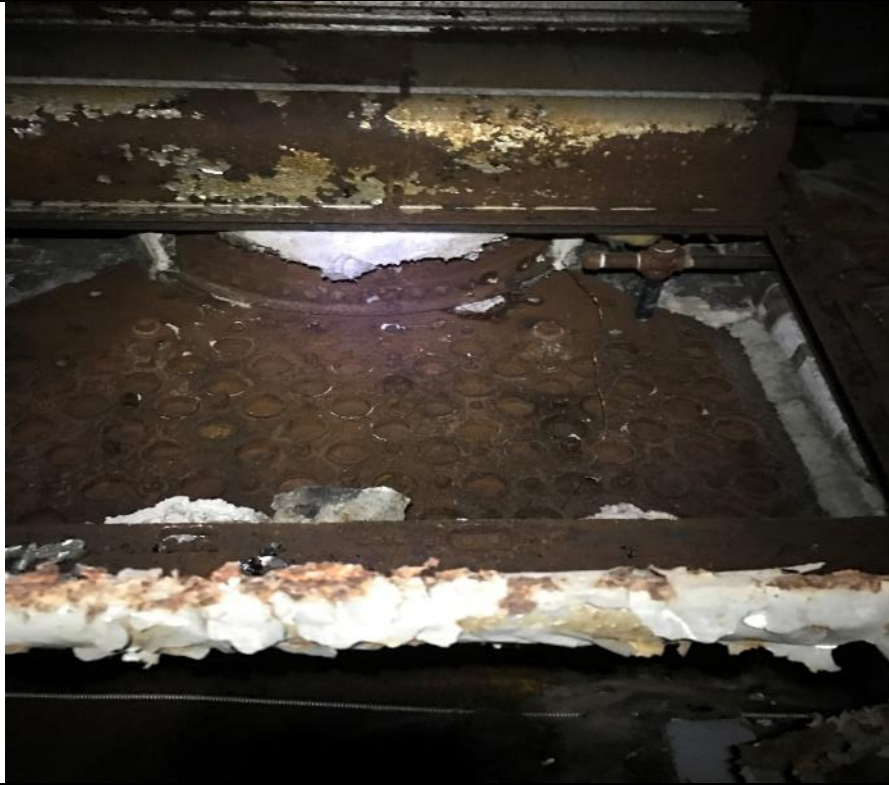
Sample 42 – 44 Boiler Insulation
