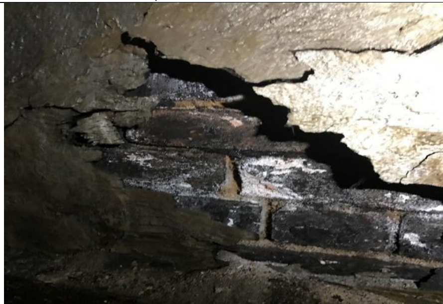
Samples 139-141 – Boiler Wrap – Tar
