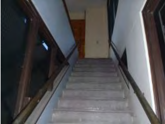
To Basement Stairwell
