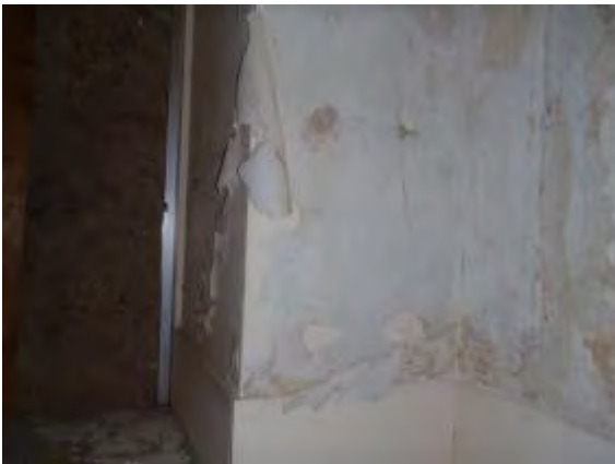
Plaster Walls Throughout
