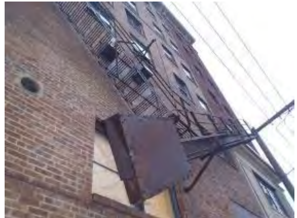
Fire Escape North Side
