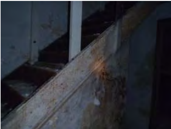
Basement-SE Stair Components
