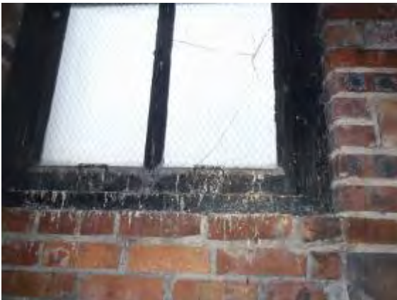
Window Components on Roof
