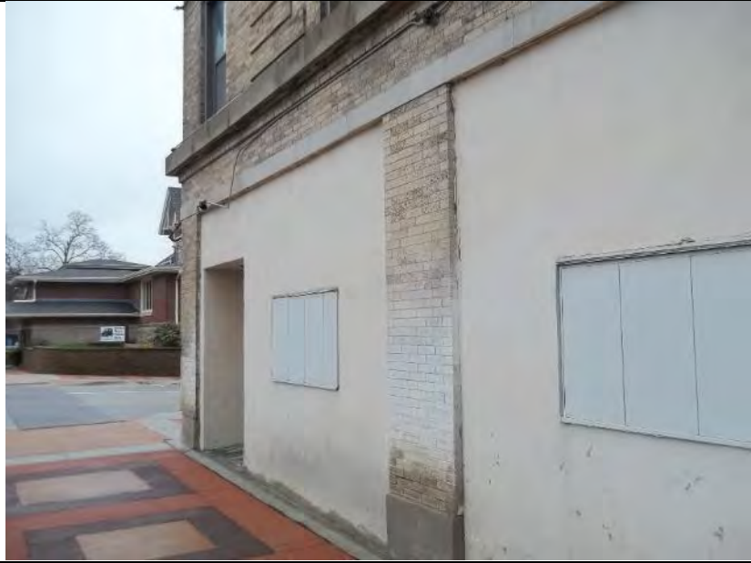
Samples 204 – Caulking around smooth stucco siding
