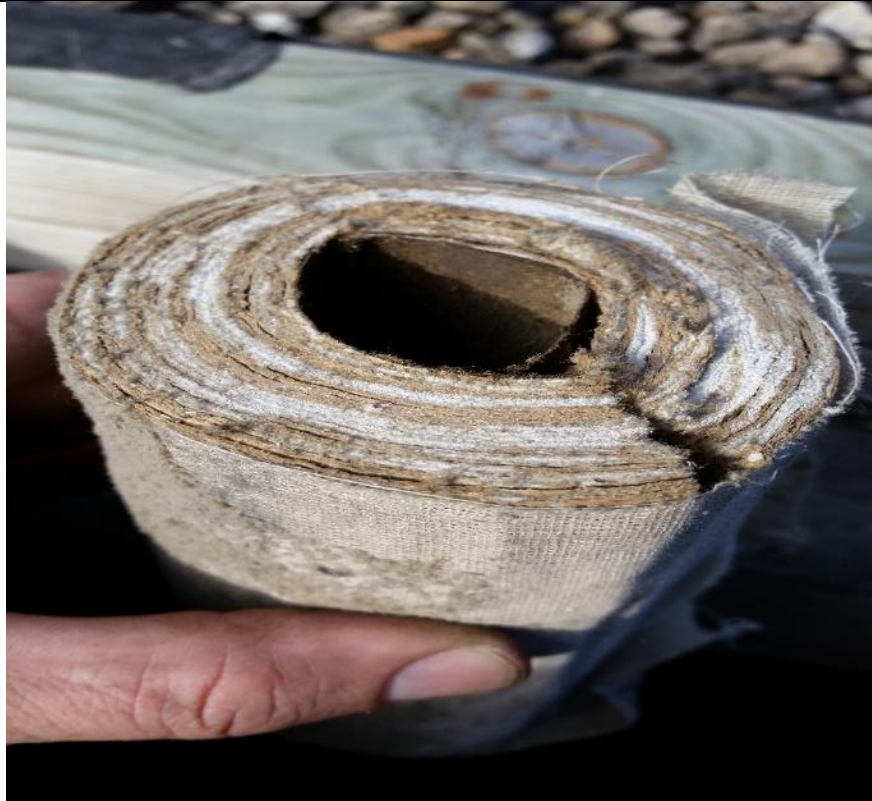
Samples 33-35 Pipe Insulation – Millboard on 1" pipes
