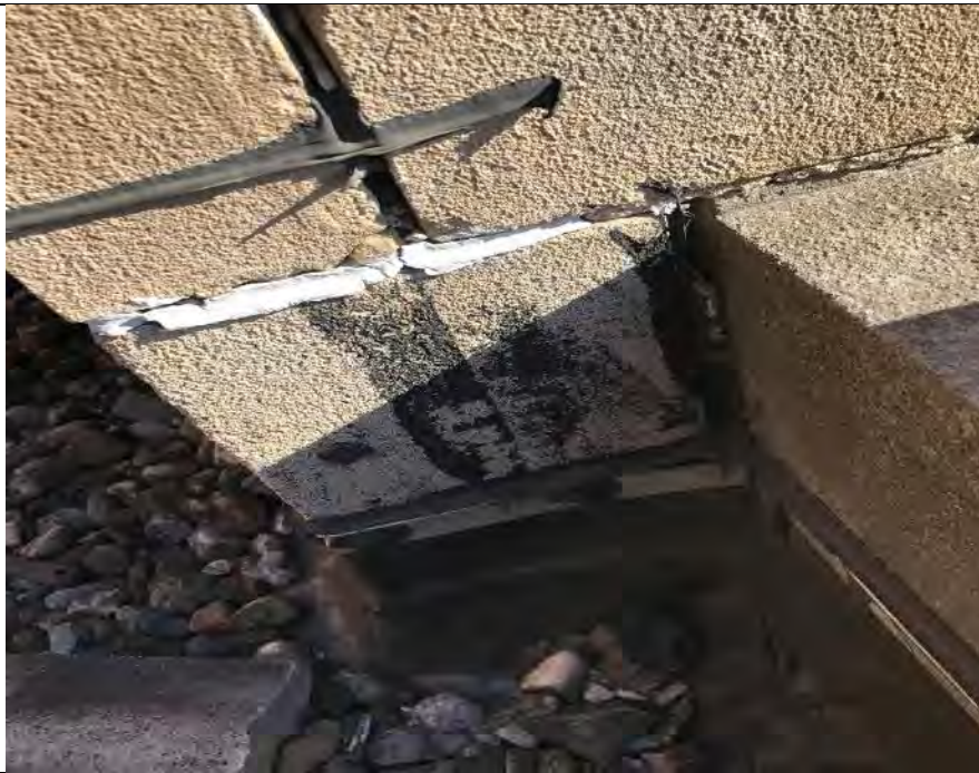
Sample 2 – White Caulking on Concrete Parapet wall – 2 nd Story Roof
