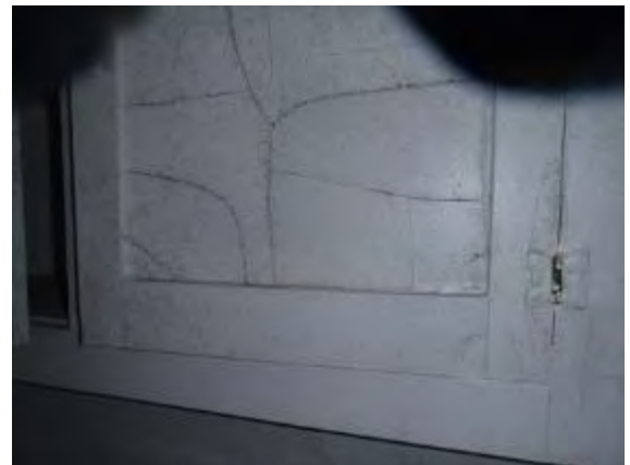
Cabinet and Cabinet Doors
