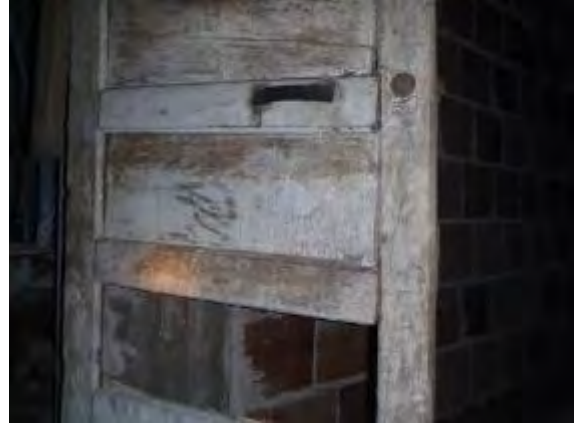
Basement-To Tunnel Door Components
