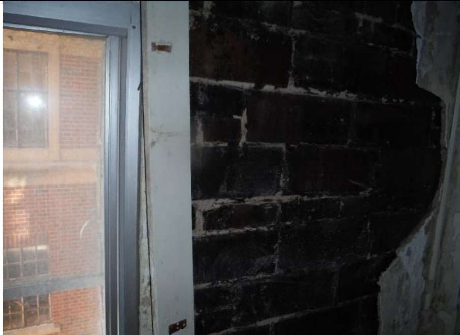
Sample 105 – Black Waterproofing on the inside of the exterior walls
