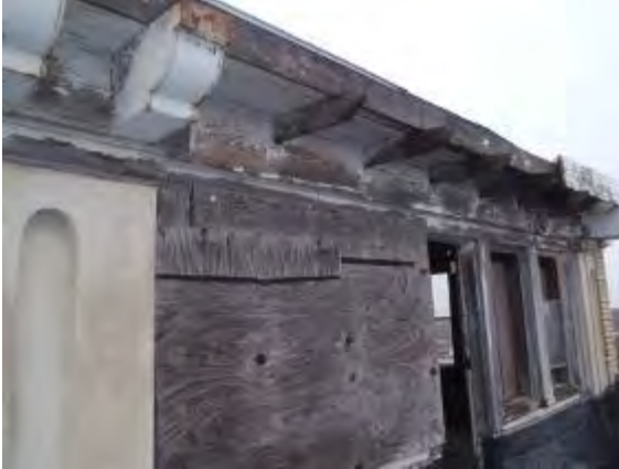
Eave/Soffit and Fascia on Roof
