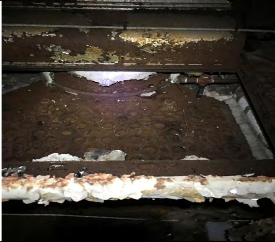
Sample 42 – 44 Boiler Insulation
